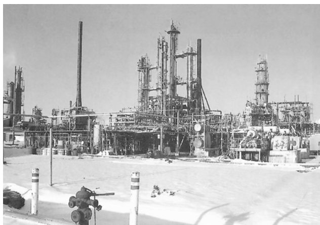
ESSO Pappas oil refinery in the industrial zone of Thessaloniki.
