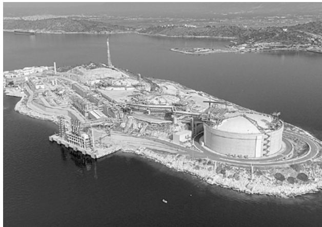
DEPA's Cryogenic (LNG) Terminal at Revythousa (1990s).
