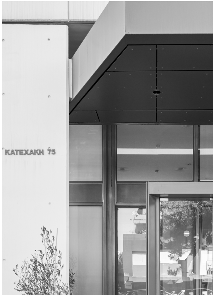
Zepos & Yannopoulos offices, 75 Katechaki avenue (Athens, 2004)
